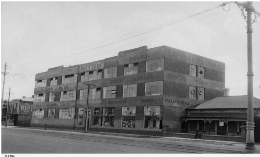
Wakefield Street [B 8184], [General description] A pair of semi-detached cottages have been demolished to make way for this addition (section of building on the right of central utility pole) to the three storey Abbott's Glassware and Paints business which was erected in 1934. The cottage on the right is for sale. Note the tram poles and wires in the foreground. [On back of photograph] 'Acre 290 / Wakefield Street, north side / 7 April 1939 / Additions made to the east side of Abbotts in 1939 / Compare with B 7219 and B 6625 / The left side of Abbott's premises abuts Daly Street, front is 49 yards'. Approximately 1939. Photographer, State Library of South Australia. Part of Acre 290 Collection.
